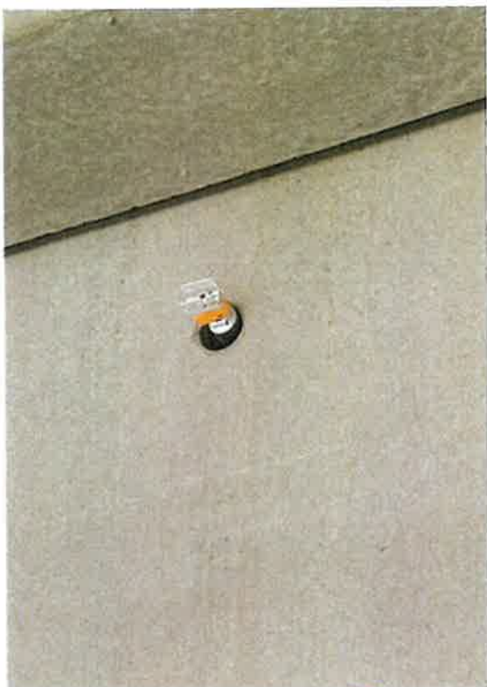
Dyse under montering
